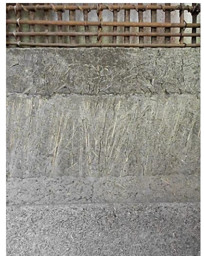
Construction of “Tsuchikabe”
