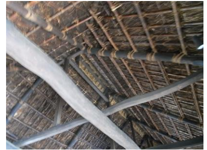
Roof seen from inside of the former Ogawa residence
