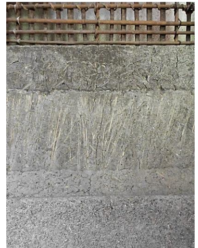
Construction of “Tsuchikabe”
